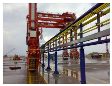
BU: Conductor bar systems supply electrical power using a current collector trolley that moves back and forth on a steel structure.
